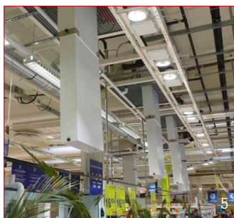
Chutes for direct filling of supermarket displays with flake ice
